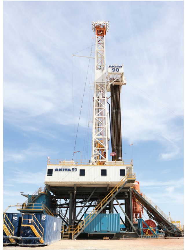
AKITA Drilling's Rig 90 is an ultrahigh-specification drilling rig operating in southeastern New Mexico. (Photo by Jennifer Presley)
